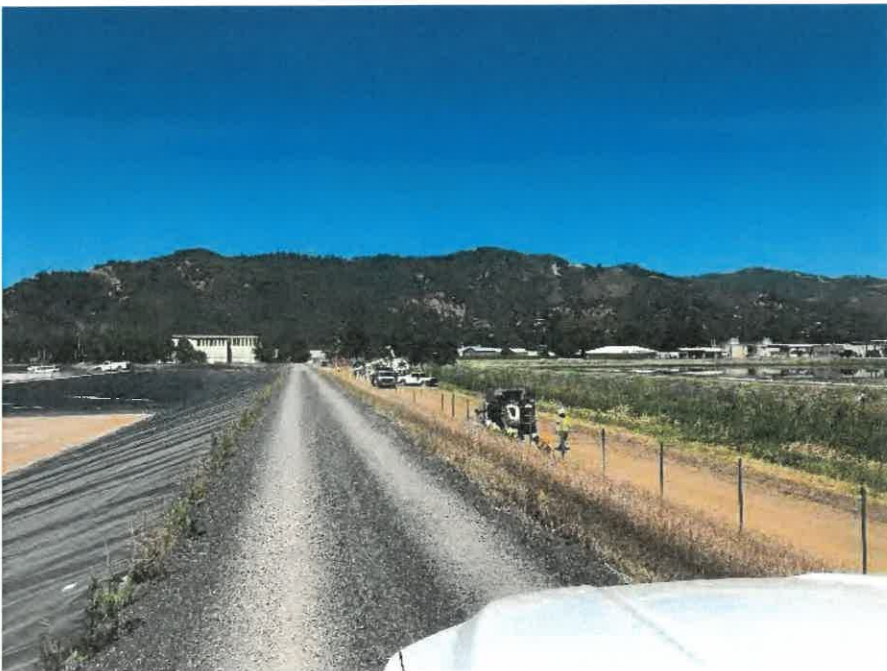
Setting fence posts at pond perimeter (6/4/19)
