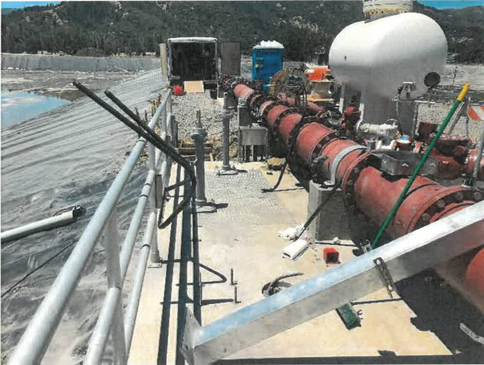
Installing conduit and wire at pond pump station (6/14/19)
