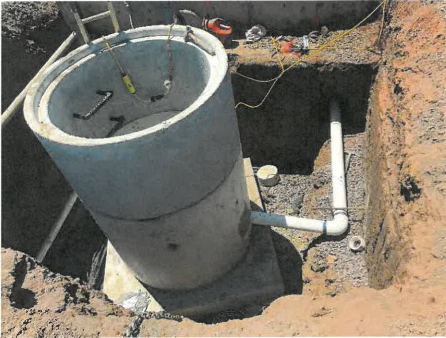
Installing generator drain manhole (6/3/19)
