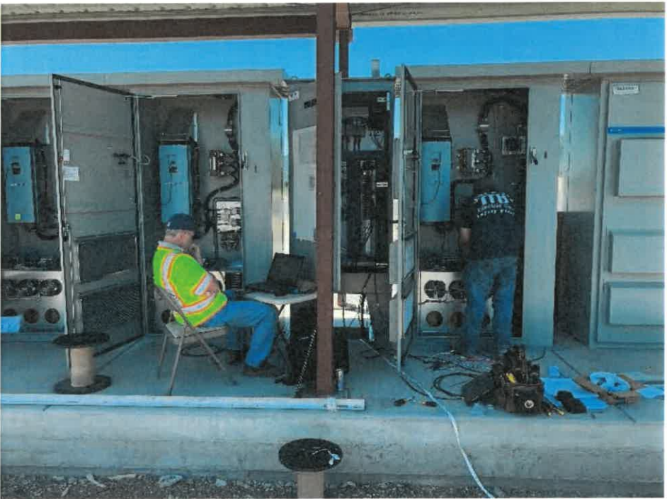
Terminating and testing fiberoptic cable at electrical panels (6/18/19)
