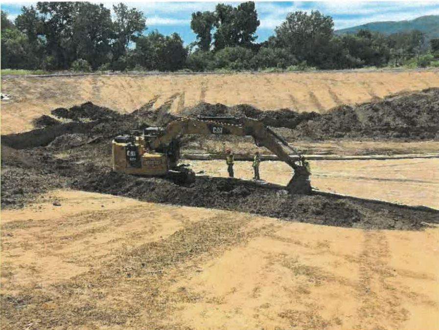
Repairing failed subgrade at Cell 2 (6/5/19)
