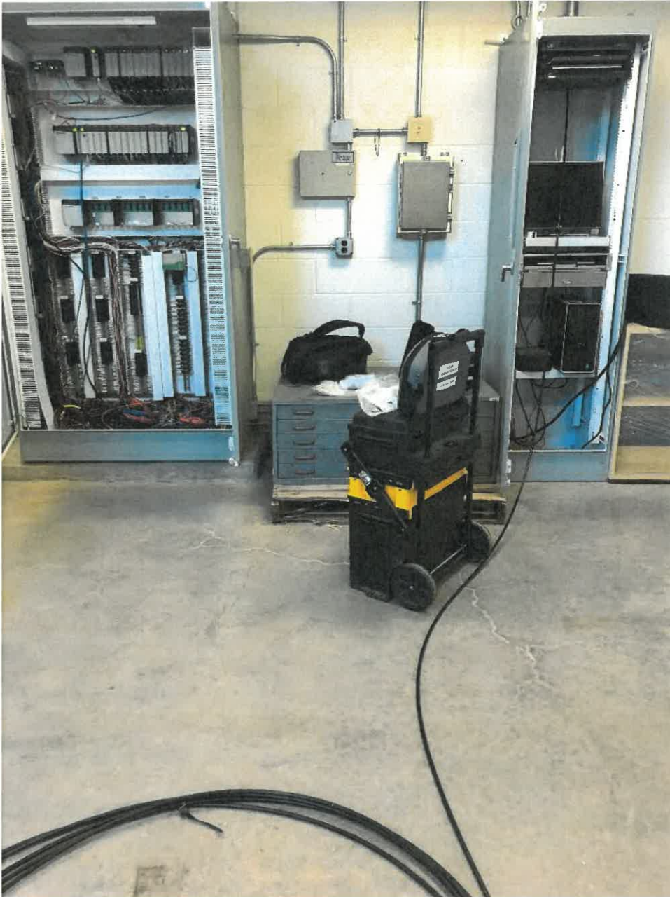
Fiberoptic cable pulled back to existing plant communication cabinet (6/18/19)
