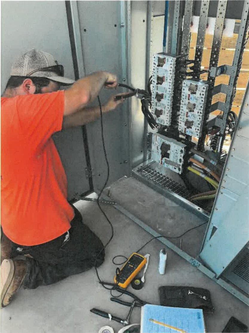
Pulling and terminating wire at pump VFDs (6/10/19)
