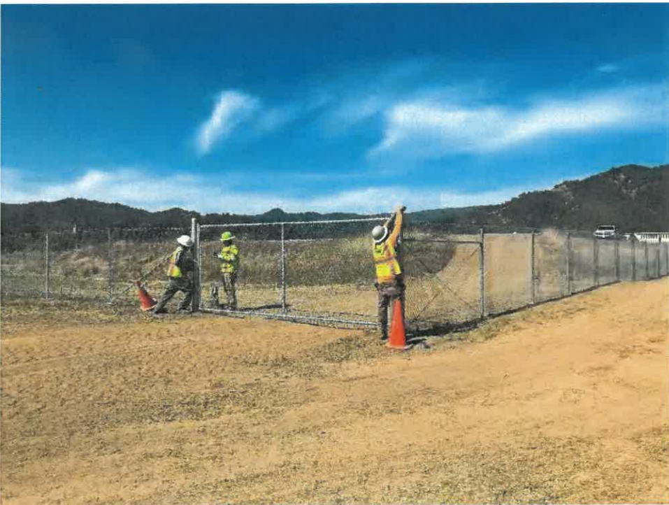
Installing gates and fence to secure facility perimeter (6/12/19)
