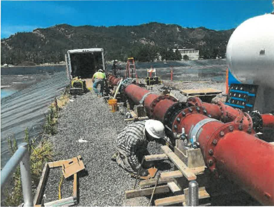
Setting up forms for pipe supports at pond pump station (6/5/19)
