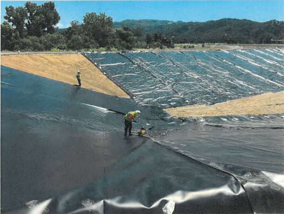
Re-installing liner after repairs to Cell 2 (6/11/19)
