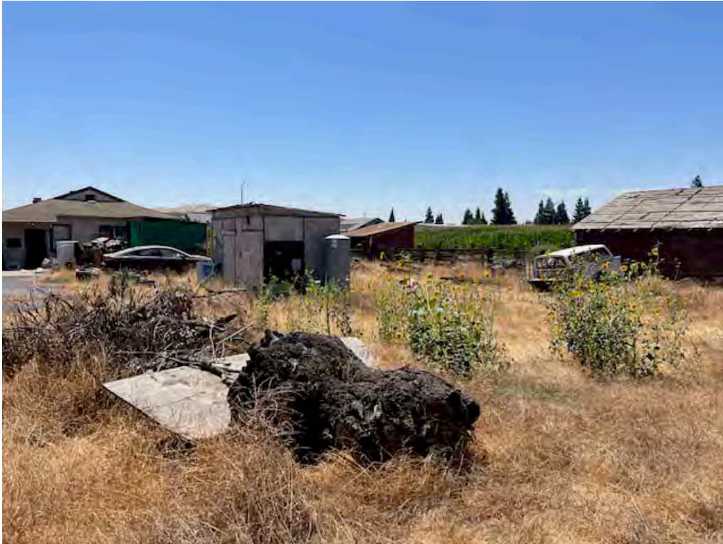
Looking SW, residence on left and 3 sheds, 8/5/2024
