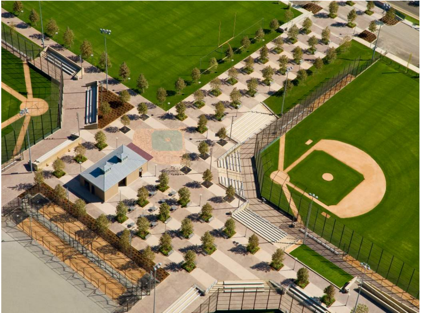
BREA SPORTS PARK. LPA, INC.
