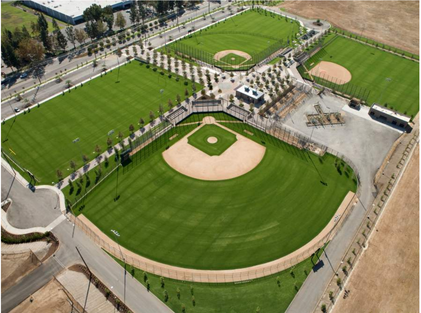
BREA SPORTS PARK. LPA, INC.
