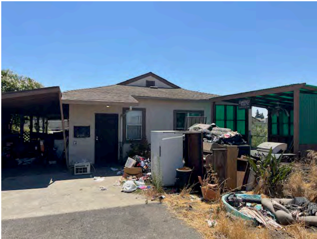
Residence looking south, 8/5/2024 note patio roof (left) is an addition.
