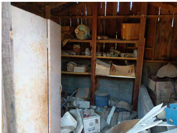
Typical interior views of the outbuildings
