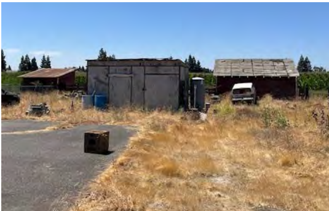
Looking west from in front of barn, 8/5/2024. Modern shed center..
