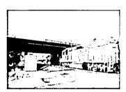
Sperry Road Extension/UPRR Grade Separation Project, City of Stockton, Stockton, California: Resident Engineer for the \$31 million project in accordance with the Caltrans Construction Manual and City of Stockton standards. The project consisted of 1 mile of new roadway alignment, two new signalized intersections, and nearly 500,000 cubic yards of imported borrow. In addition to the roadway items, four new bridge structures including one over an environmentally sensitive creek and three
